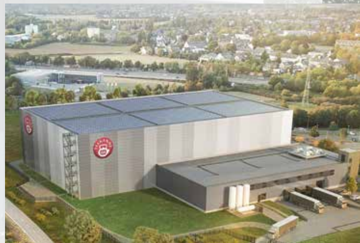
This is what the TEEKANNE Tea Processing Centre will look like one day.
